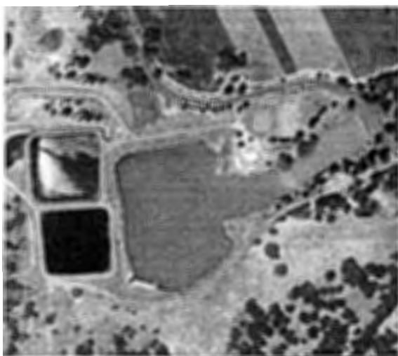
View of the WWTP and Algae in Storage Pond
