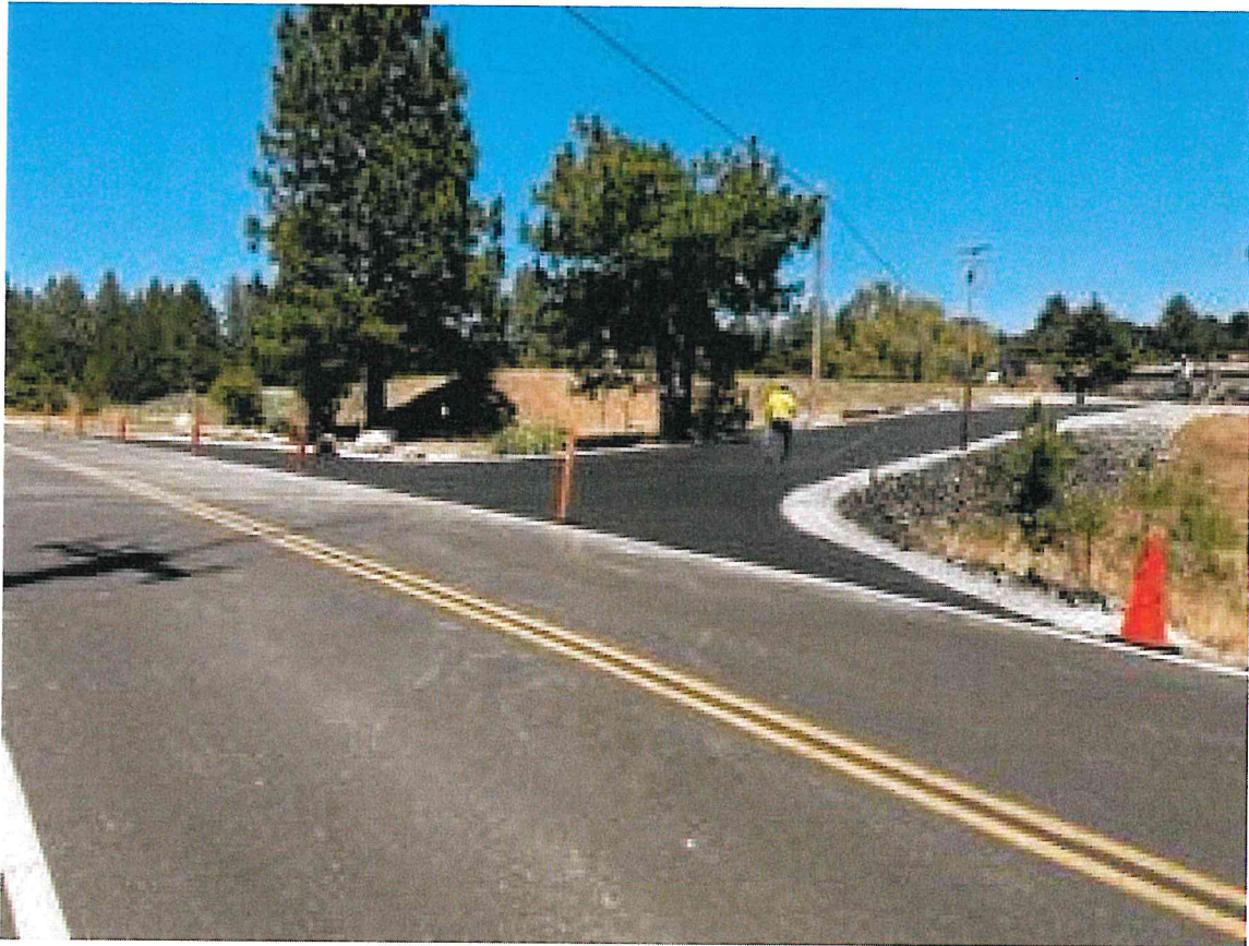
Road base, riprap and grading installed and compacted 6/28
