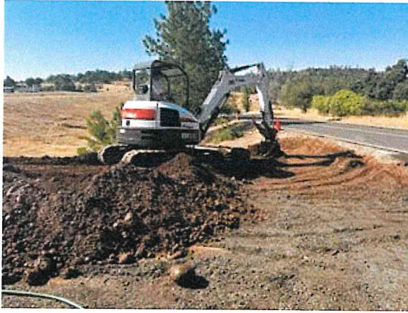
Road base, riprap and grading installed and compacted 6/28
