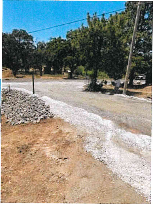
Road base, riprap and grading installed and compacted 6/28
