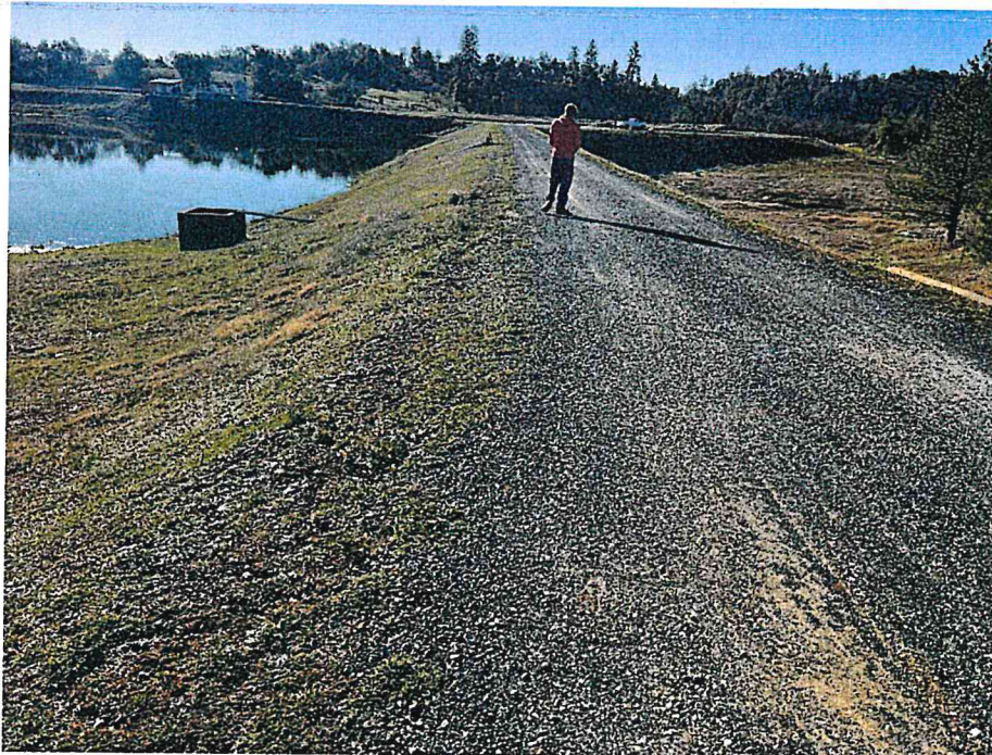
1. Upstream face of west dike with good vegetation control.
