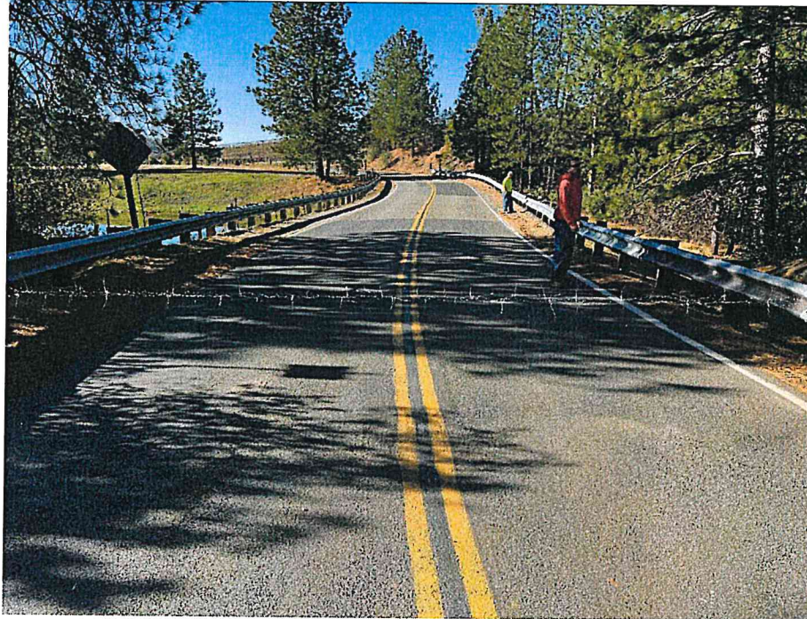
8. Main Dam crest observed from right side.
